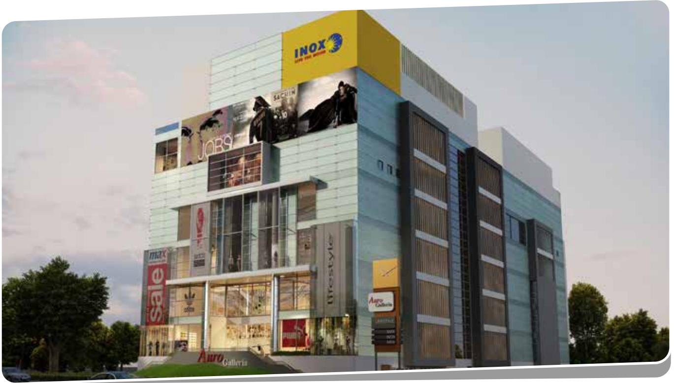
Client : Assam Tea Warehousing | Total Area : 2,20,000 sqft | Location : Dispur, Guwahati
