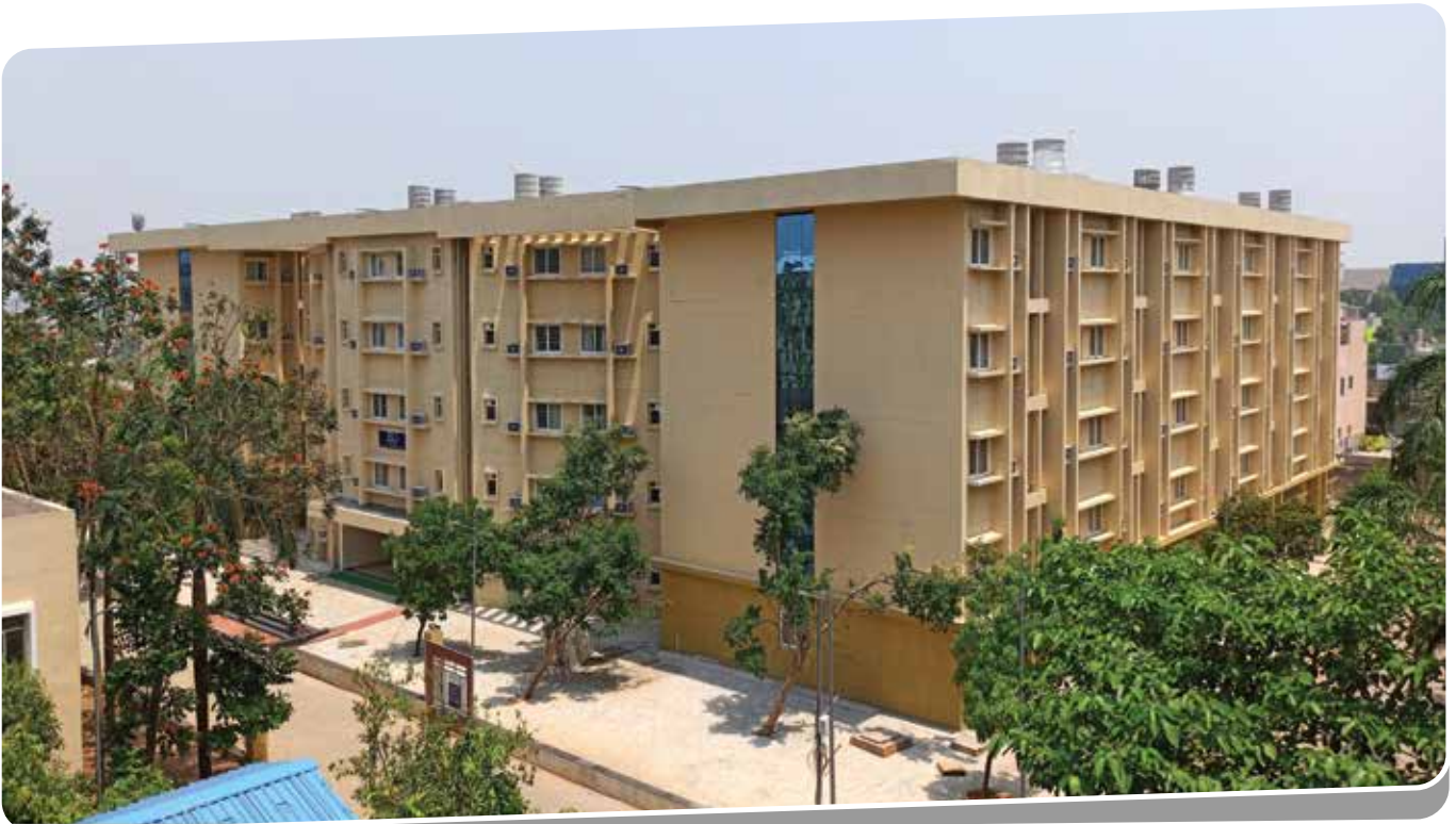
Client : Kalinga Institute of Industrial Technology | Total Area : 1,50,000 sqft | Location : KIIT Campus, Patia, Bhubaneswar
