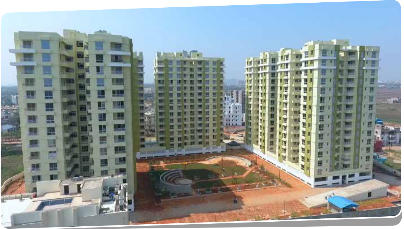
Client : Sri Jagannath Promoters and Builders | Total Area : 5,25,000 sqft | Location : Shani Mandir, Khandigiri, Bhubaneswar
