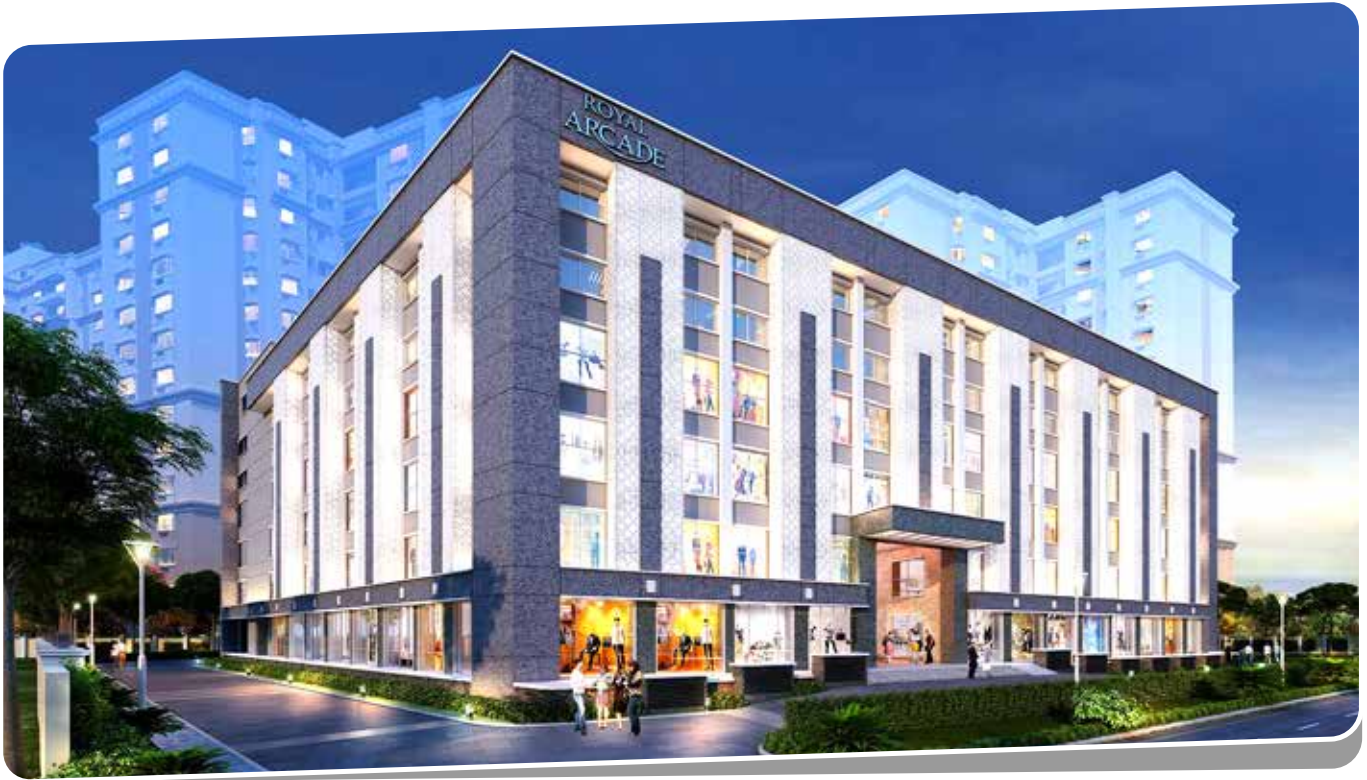
Client : Ashiana Homes Pvt. Ltd. | Total Area : 2,50,000 sqft | Location : Nandankanan Road, Raghunathpur, Bhubaneswar
