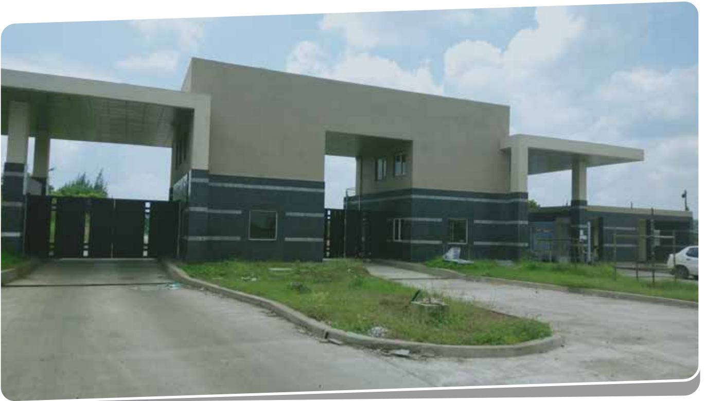
Client : MGM Minerals Limited | Total Area : 1,20,000 sqft | Location : Dhenkanal, Odisha
