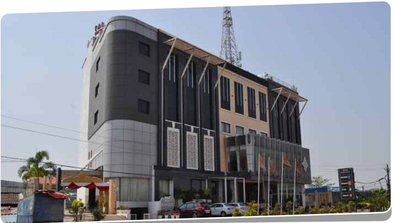
Client : Mr. Satpal Singh, Pal Heights | Total Area : 1,20,000 sqft | Location : Hotel Pal Mantra, Pahal, Bhubaneswar
