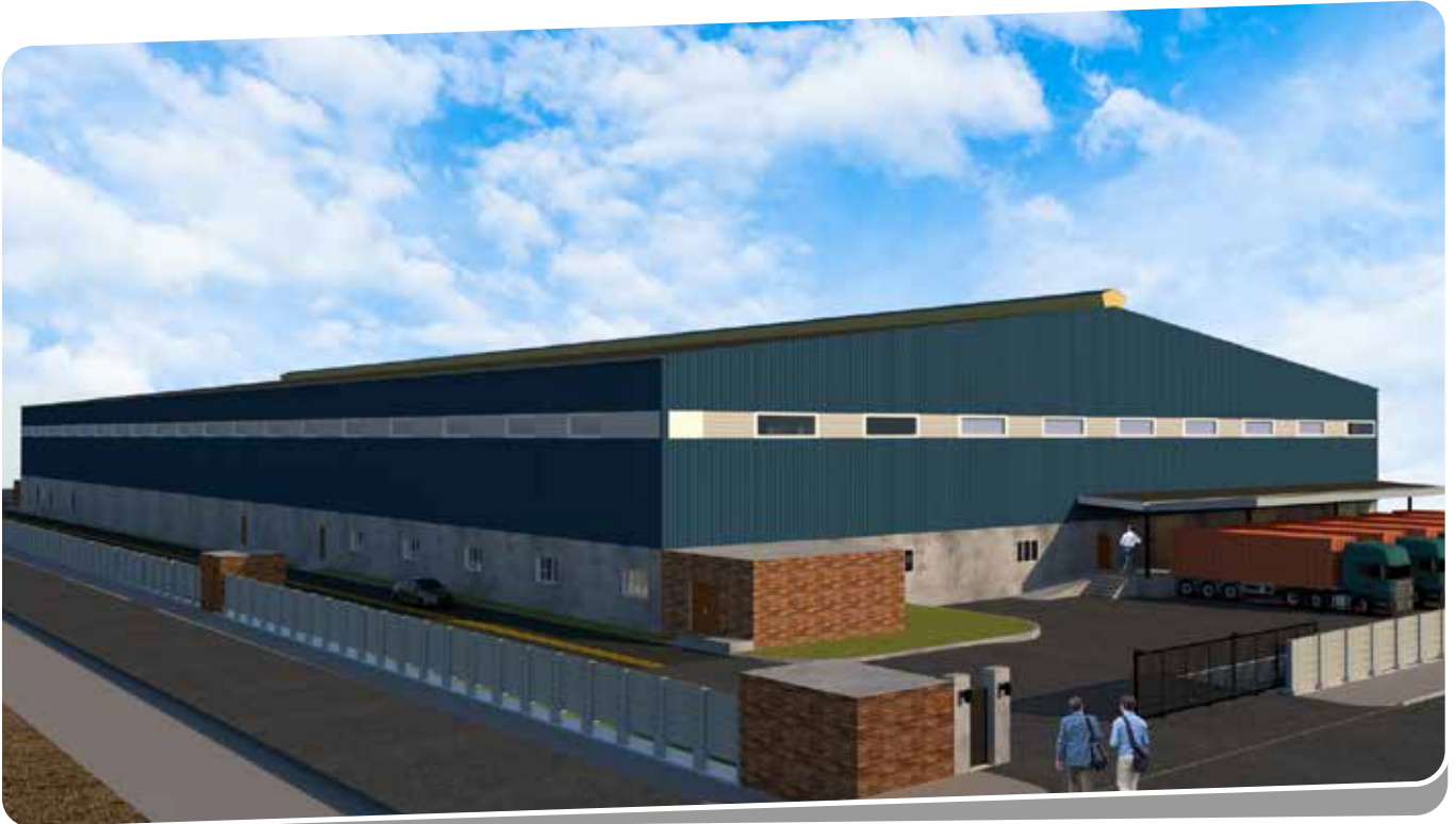
Client : Jubilee Bottlers Pvt. Ltd. | Total Area : 1,00,000 sqft | Location : Chhatabar Industrial Estate, Khorda
