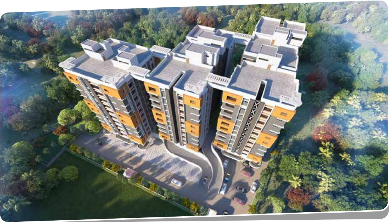
Client : Balaji Builders & Developers | Total Area : 3,03,641 sqft | Location : Tangarpali, Ainthapali, Sambalpur Town Unit-15
